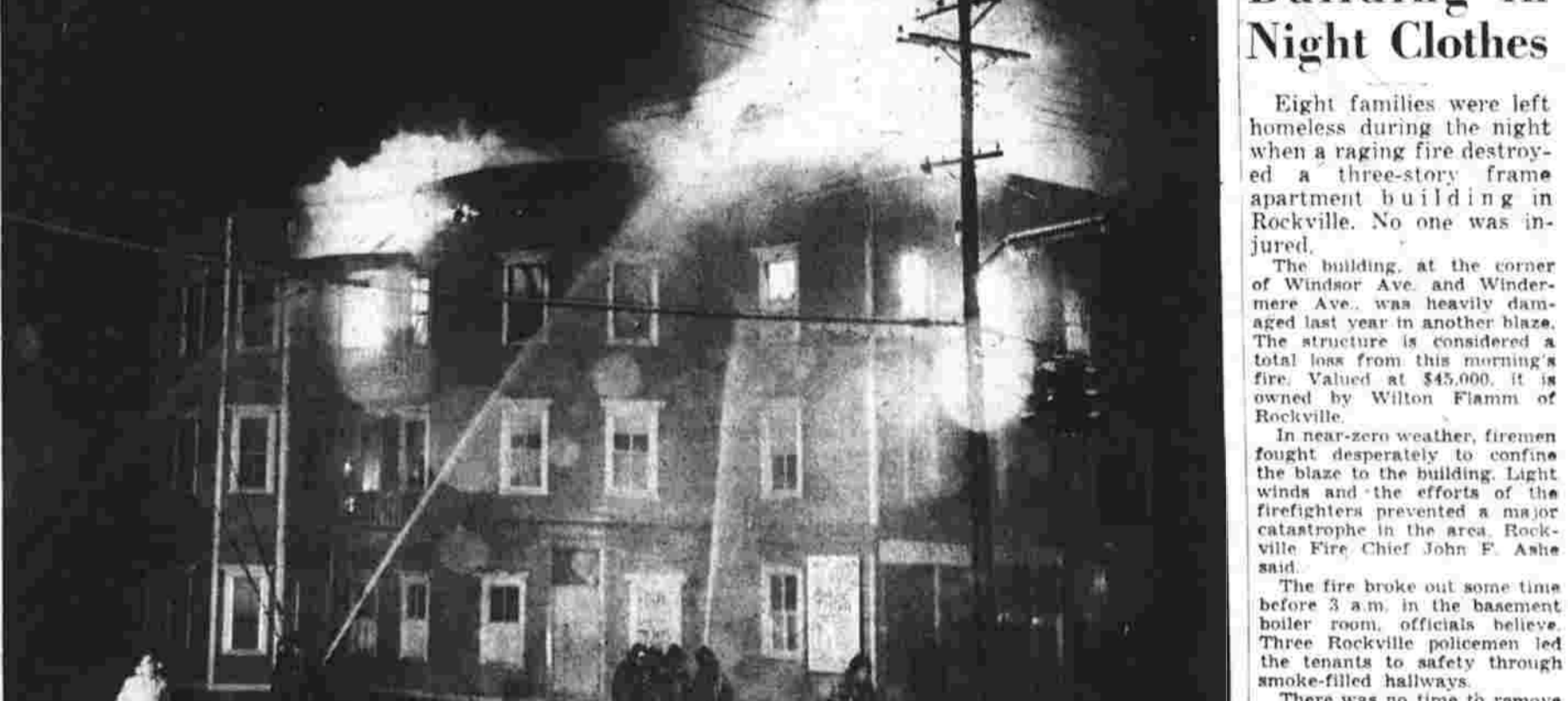
Flames break through the roof of the Flamm building in Rockville today. (Herald photo by Saterini.)
